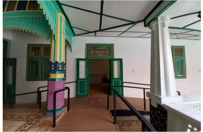
Picture 10. Ramp facility for accessibility Doc. Kanisa Triyundari Arselant, 2023
